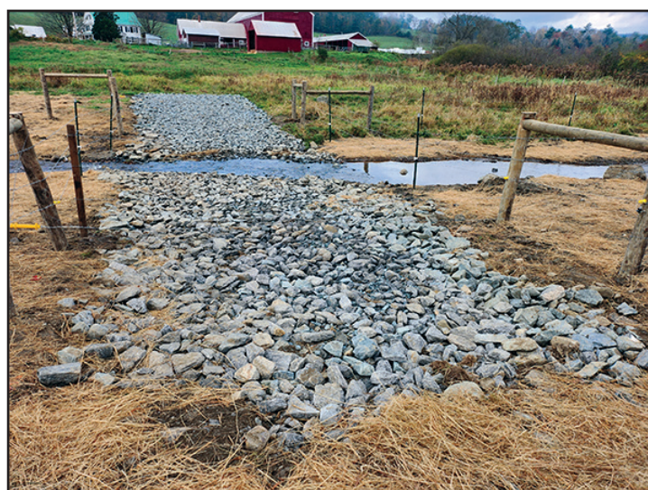
Cattle crossing protects stream from sedimentation.
